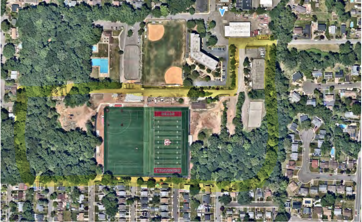
19 - This is an up to date aerial of what the site looks like after two initial phases of redevelopment.
