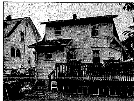
REAR (NORTH) VIEW OF HOUSE
